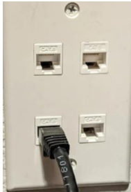
Ethernet Port in Wall
